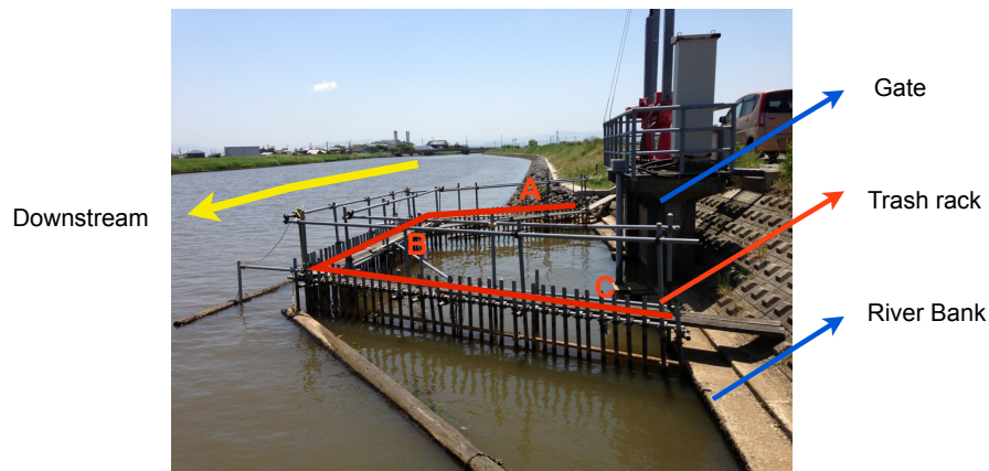
Fig. 5-9 The inlet at Nagasai intake pumping station
