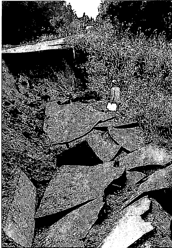
写真-1 20mにわたり陥没した鯖石川ダム右岸の町道(田代地区) Photo 1 Rode seriously collapsed for 20 m by the main shock in the right bank of the Sbaishi-gawa Dam, Tashiro, Taka- yanagi-machi, 6 km SE of the epicenter.
