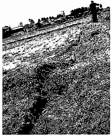
Photo 4 Straight crack 620m long appeared in the paddy field of the epicentral area, Kamitakada, Sasakami Village.
