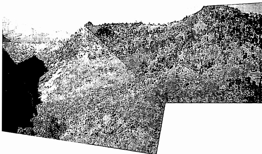
**Photo 6** : Landslide at Sidhartha Highway that was induced due to road excavation at old sliding area
