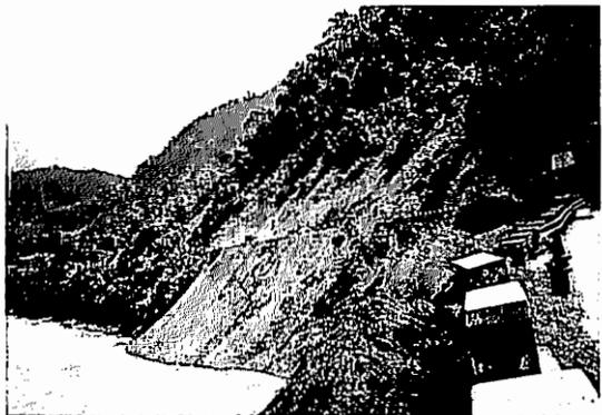
Photo 3 : View of Dahakibhir landslide, a recent problem to the Prithvi Highway.
