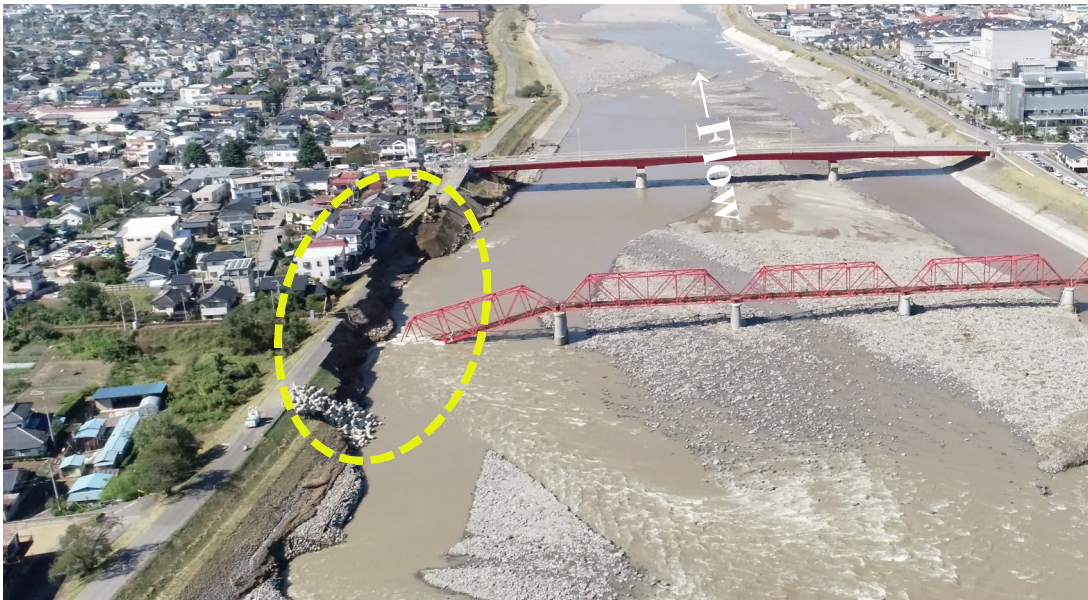
Figure 1.2: Aerial photos of The fall of Ueda Bridge in Chikuma River of the Japan
