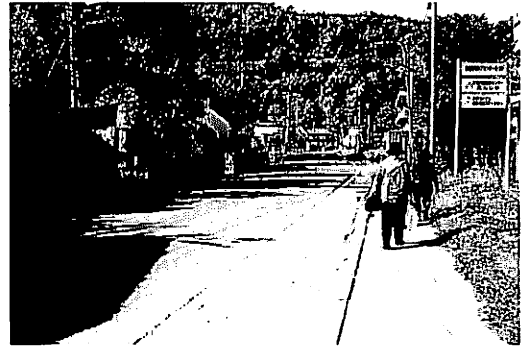
Photo 11 : Deflection in the road after the movement of the ground (can be noticed from the deflected road marking)
