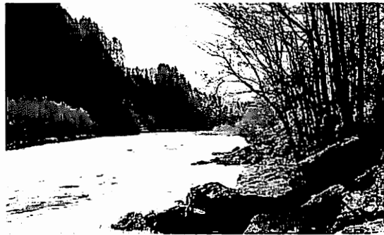
写真-20 Iller川の近自然河川改修状況 (巨礫を用いた水制工) Photo.20 Natural river restration of Iller river (Spur dyke constructed withbig stones)
